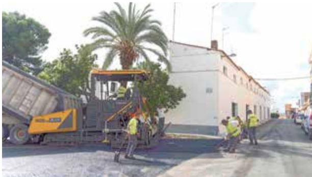
Treballs a Picassent. / EPDA
