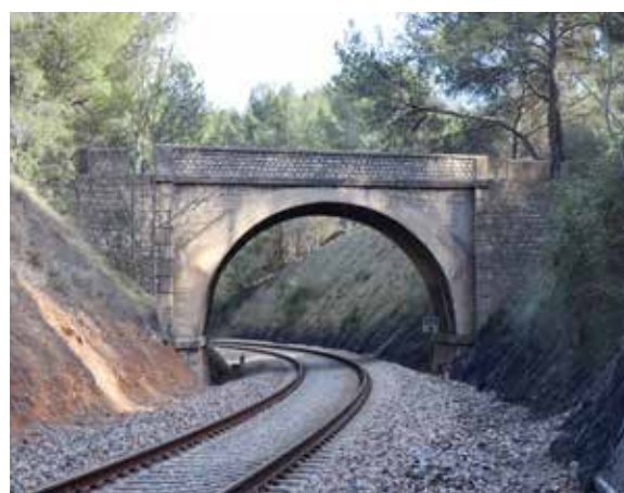
Navajas km 232+397 Paso carretera CV-213./ EPDA
